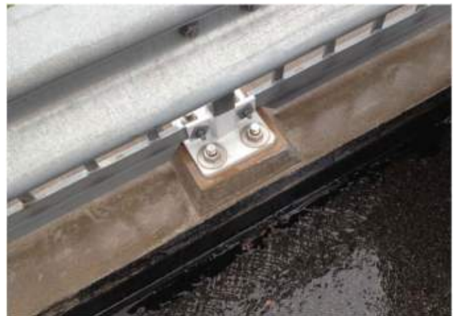
Figure 1. A replaced BEBS in a bridge in the south-west of Sweden.
