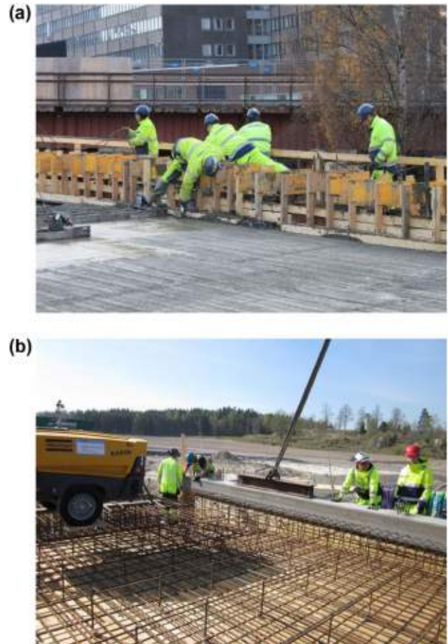
Figure 4. Edge beam construction in real bridge projects: (a) type I, and (b) type IV. Source: Kelindeman (2014).
